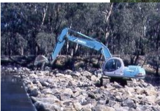
Above: A Water and Rivers Commission contractor undertaking repairs on the Extracts Weir. This work was to stabilise rock movement- this demonstrates the power of water flow.
